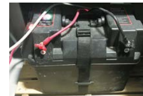
蓄電池 12V Storage battery 12 V
